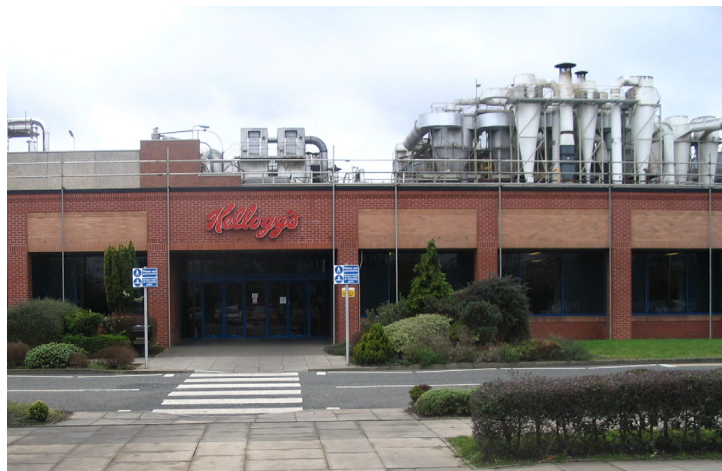
Kellogg snack plant in Wrexham, Wales
